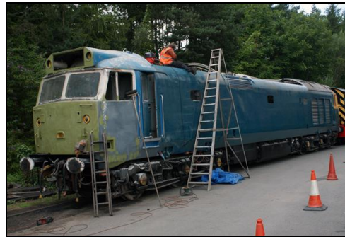
Restoration work in progress at Buckfastleigh
